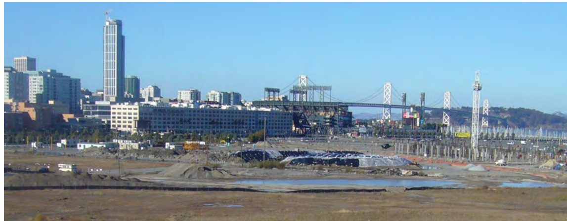
Construction work at Mission Bay UCSF Campus as of October 2007
